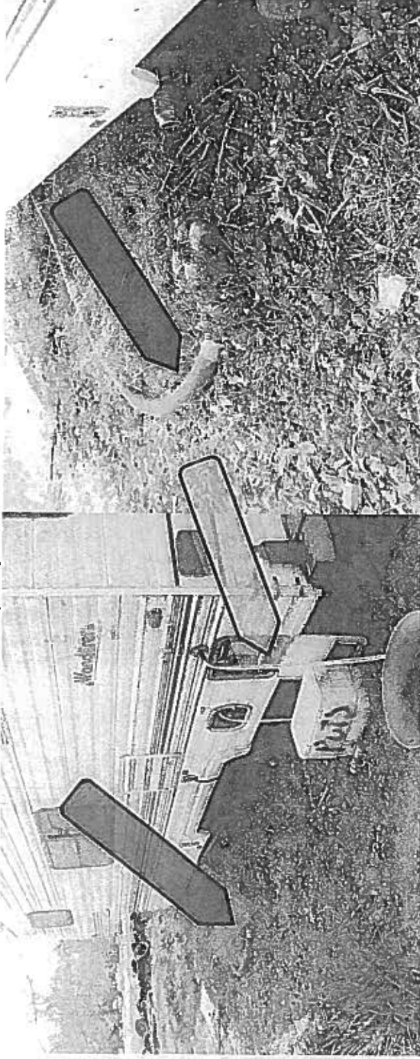
Pictures showing travel trailer sewer line (red arrows) not attached to proper sewage system and water line hook up (yellow) indicating occupancy of trailer.
