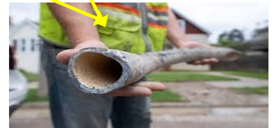
Lead Service Line
